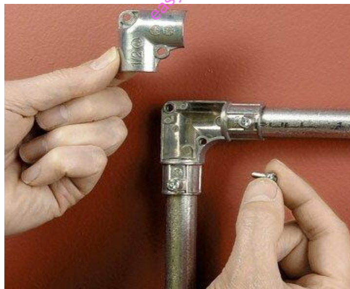
Figure 38: Additional Step to Install a Pulling Elbow
