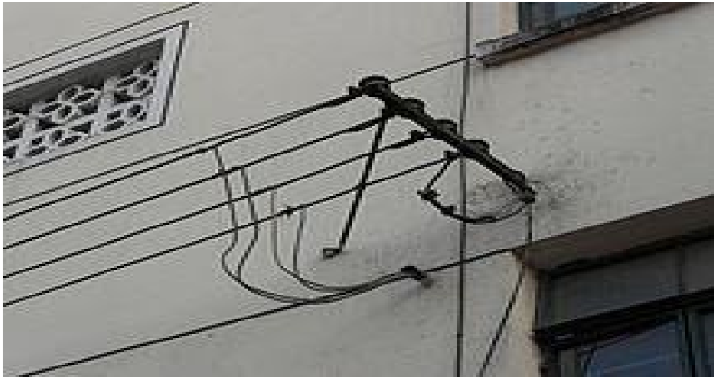
Figure 18: House Service Overhead System
