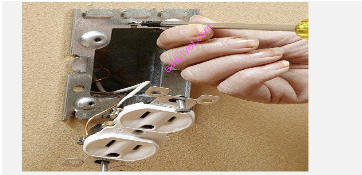
Figure 46: Step, Install Raceway Starter Box
