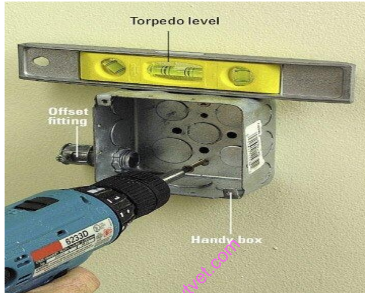
Figure 33: Step 1, Anchor Boxes
