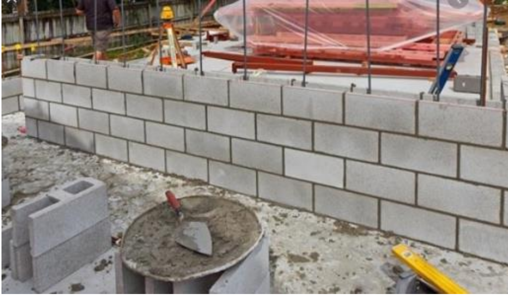
Figure 168: Constructing masonry block wall
