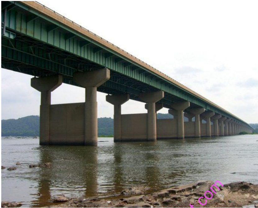
Figure 127: Example of a bridge, Nyali Bridge
