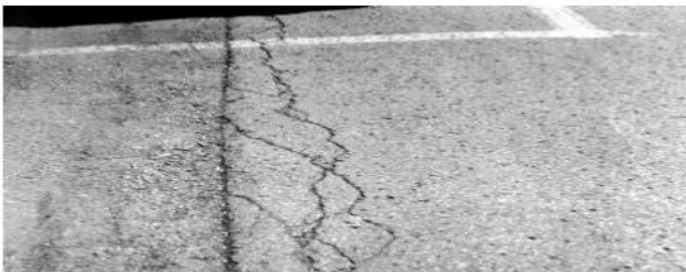
Figure 142: Edge cracking
