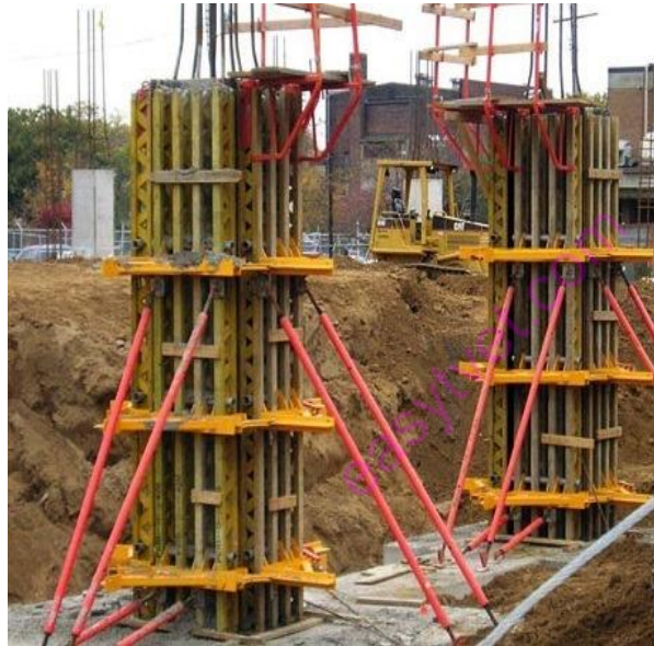
Figure 14; Column formwork
