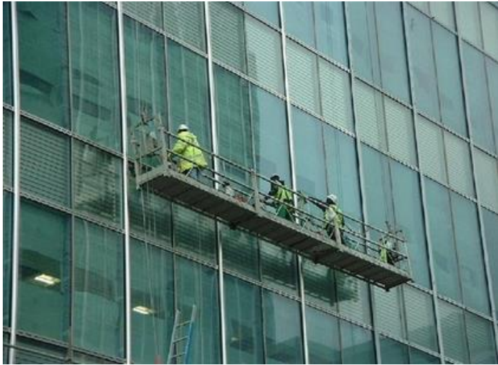
Figure 28: suspended scaffolds
