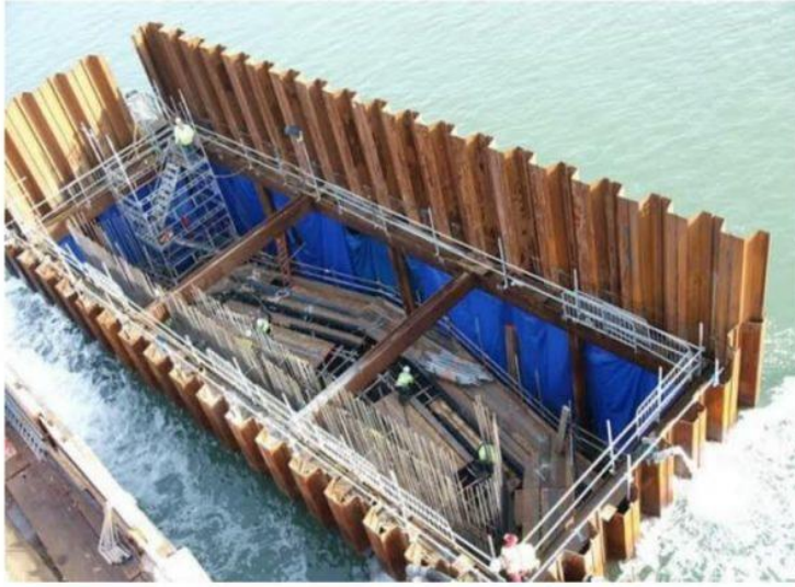
Figure 11; sheet piling
