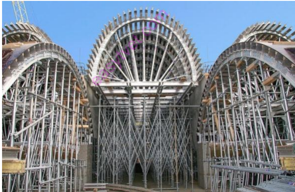
Figure 19; example of special formwork
