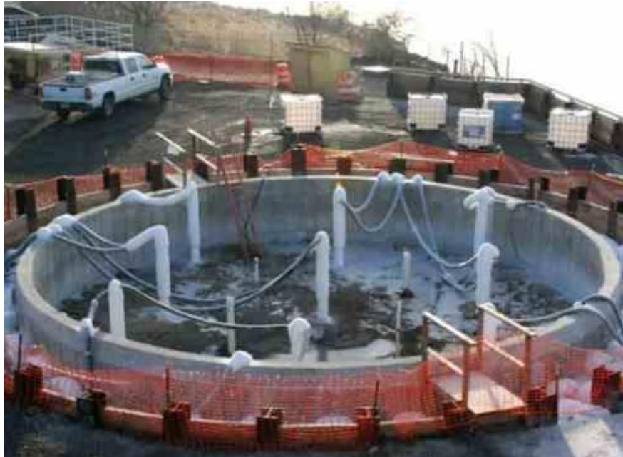
Fig. 40 Ground freezing
